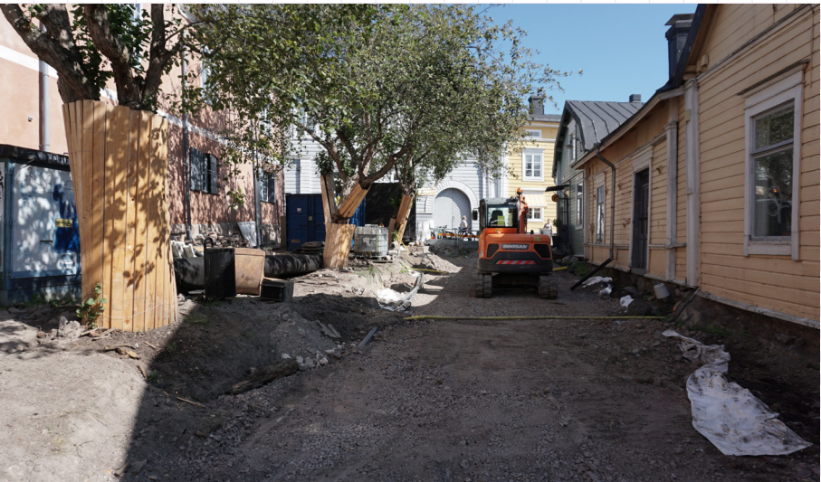
38 It is necessary to pay special attention to the protection of trees during construction work. It is vital to protect the tree trunks from mechanical damage by wood-wrapping and to secure the protection of root systems during construction. Porvoo, Finland
