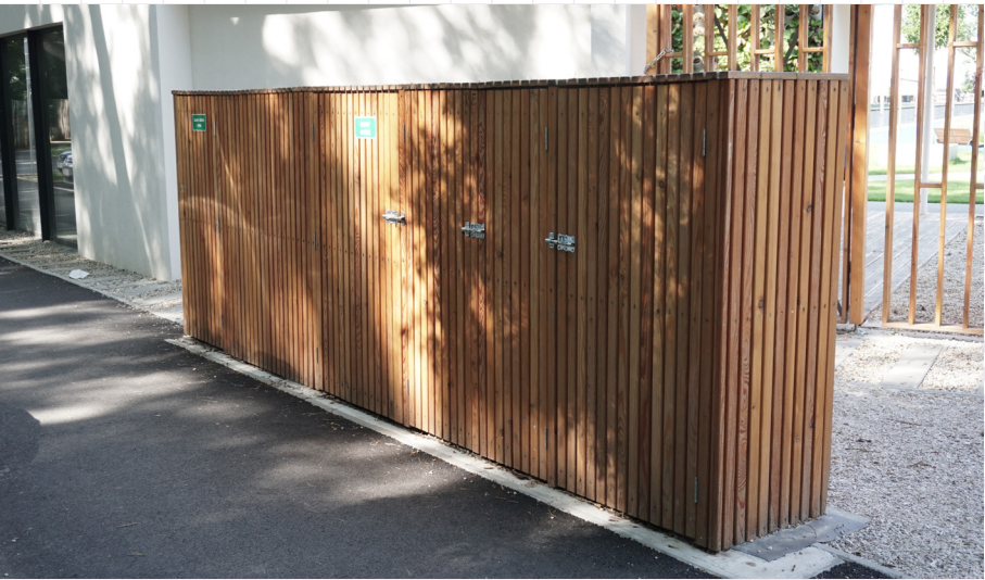
40 A good example of merging above-ground engineering networks in a way that reflects on the visual identity of a public space. Bratislava, Jama Park
