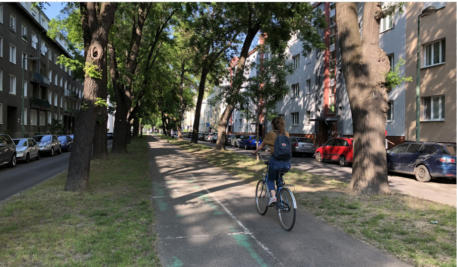
14 An apt solution for a safe and segregated bike path, which is guided separately through the middle of a traffic-calmed street and separated from individual and pedestrian traffic. The tree alley also offers cyclists climatic comfort. Bratislava, Trenčianska Street
