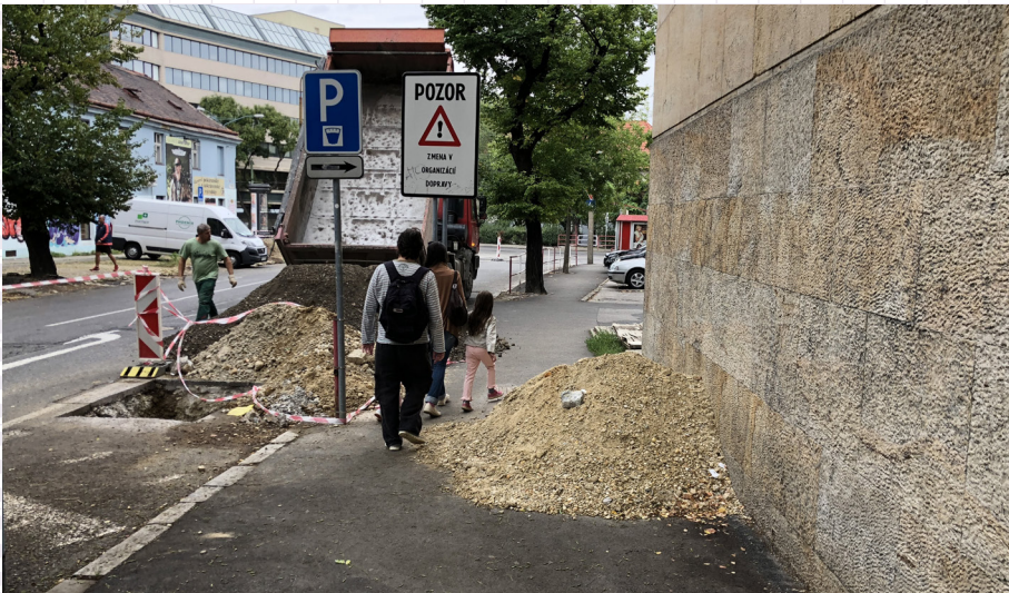
35 Incorrect marking, enclosing or overt narrowing of the direct pedestrian lane is unacceptable during construction and repair of public spaces. Bratislava, Vazovova Street
