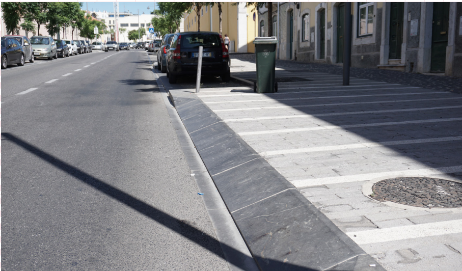
31 A suitable approach to surface solutions in public space is a choice of high-quality, lasting, and replaceable surfaces ideally acquired from local sources. It is necessary to design edges and boundaries with a considerations of potential car traffic stress. Lisbon, Portugal
